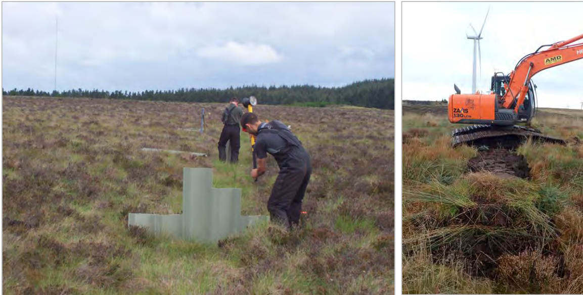
Photos 10 & 11: Plastic piling (left) and conventional peat dam mid construction (right)
