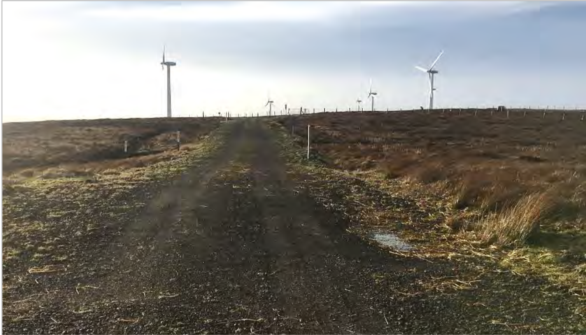
Photo 12: Road leading to T10 proposed to be decommissioned and restored
