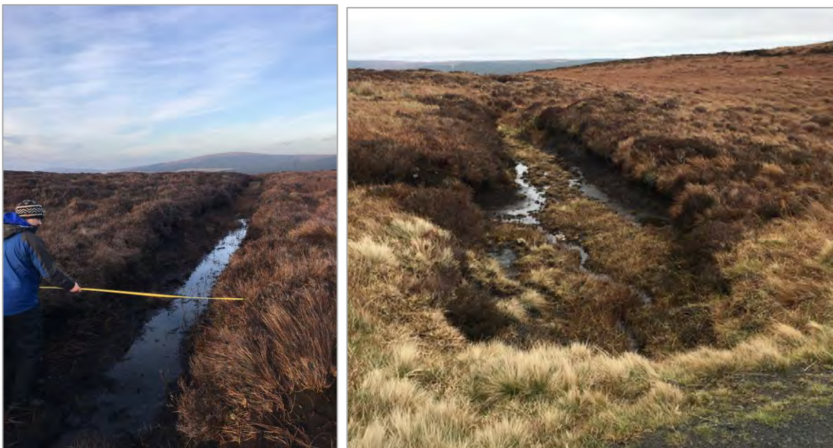
Photos 3 & 4: Two of the large drains bordering Unit B
