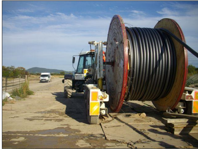
Plate 5.4: Typical Tractor and Trailer Set-up for Cable Drum Transportation 5
