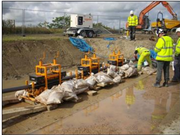
Plate 5.5: Jointing bay Layout and Cable Pulling 6
