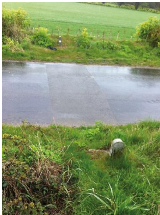
Plate 5.7 A buried cable road crossing One to Two years After Construction. 9
