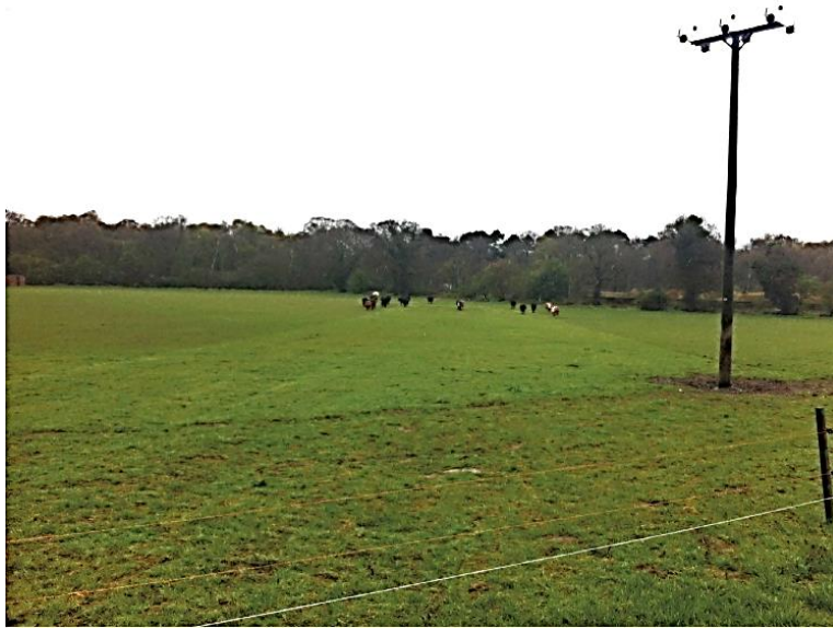
Plate 5.6 A Buried Cable One to Two Years After Construction 8
