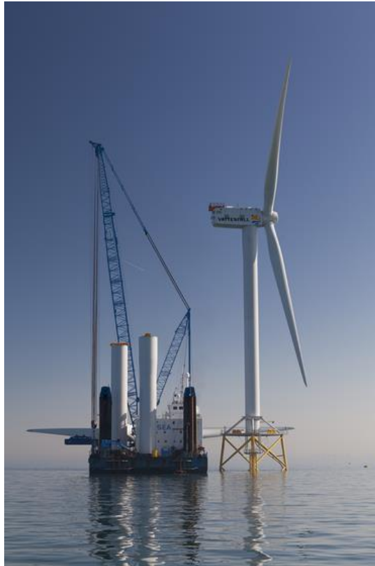
Plate 5.3 Wind Turbine Under Construction 3
