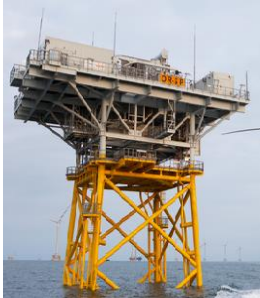
Plate 5.1 Typical offshore AC Collector Station 1
