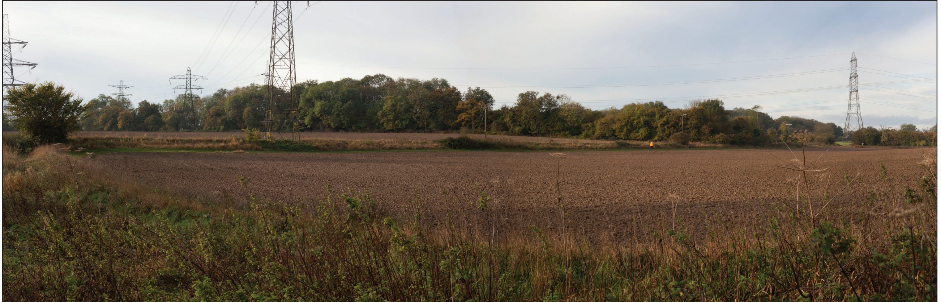
Photomontage View of East Anglia THREE Phase 1 substation with East Anglia ONE converter station (only visible features are labelled).
