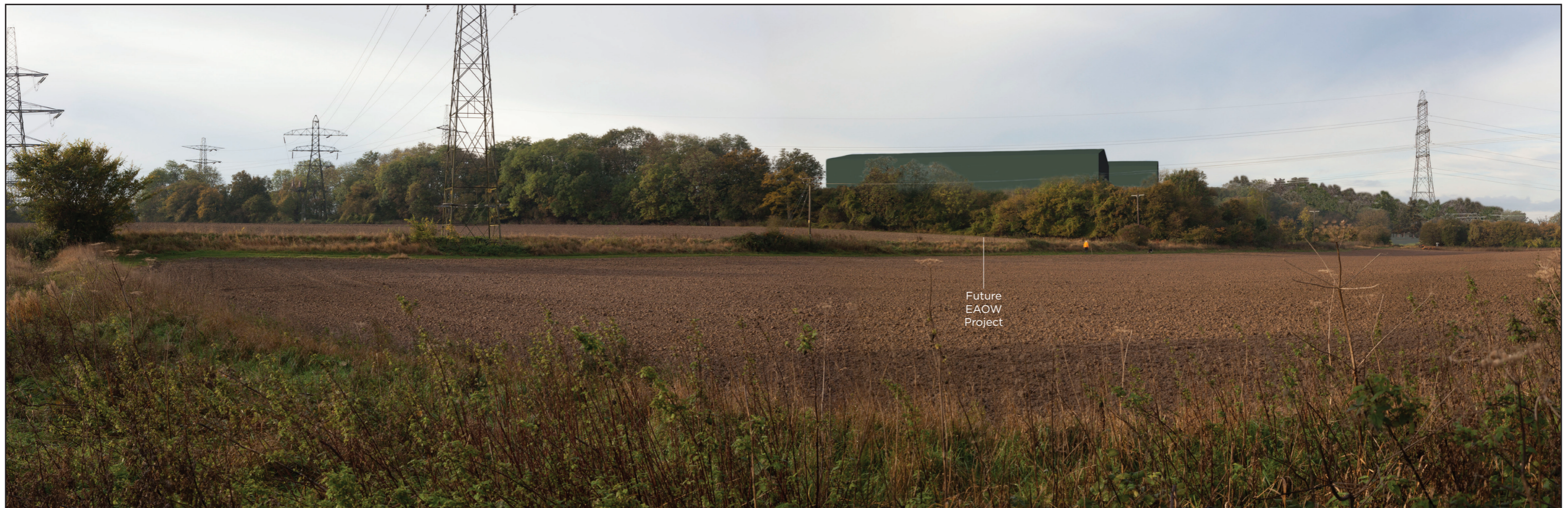
Photomontage View of East Anglia ONE converter station, East Anglia THREE substation and a future EAOW project with landscape mitigation (only visible features are labelled).
