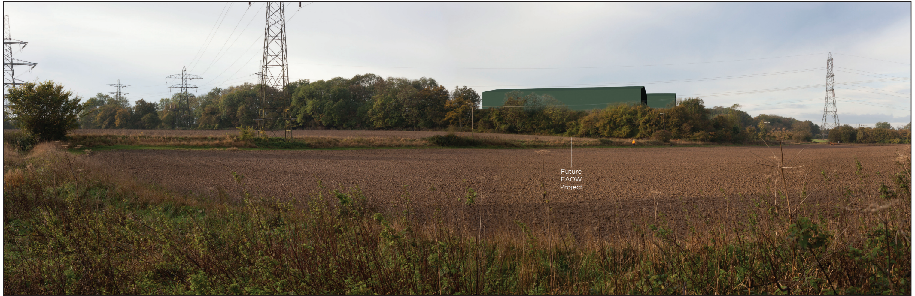
Photomontage View of East Anglia ONE converter station, East Anglia THREE substation and a future EAOW project (only visible features are labelled).
