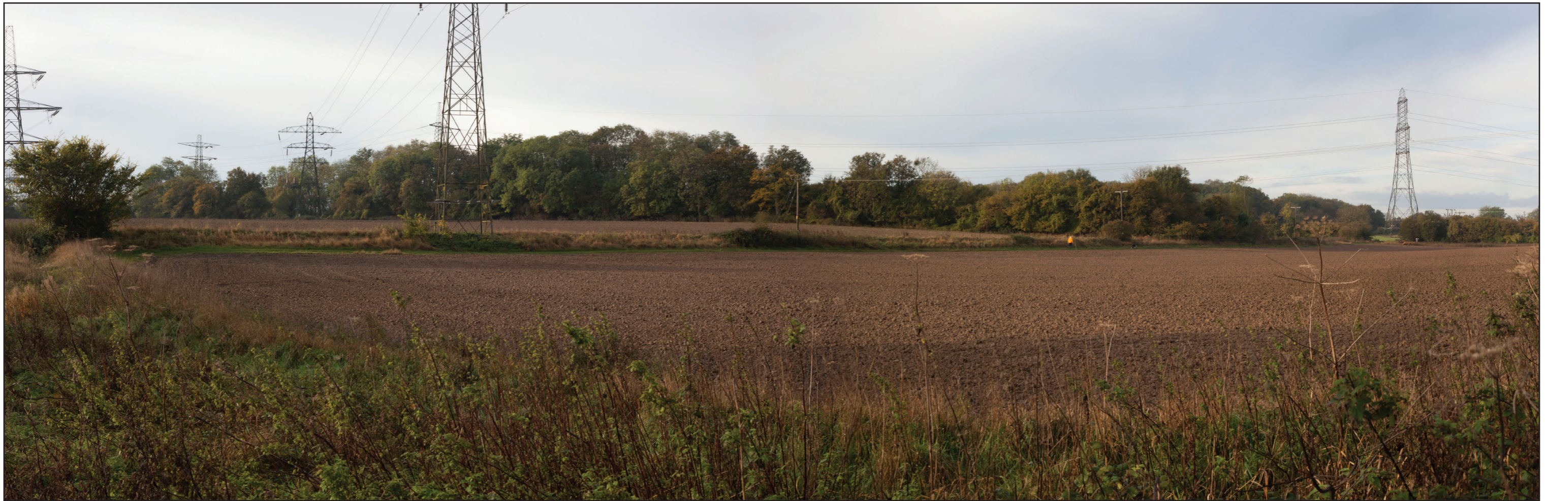
Photomontage View of East Anglia THREE Phase 2 substation with East Anglia ONE converter station (only visible features are labelled).
