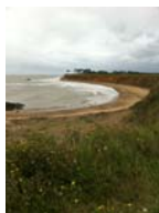
EAOW Intertidal North W2 - coastal erosion 1
