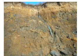
EAOW Intertidal North W31 - erosion + FW input 1
