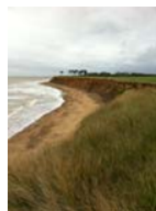
EAOW Intertidal North W2 - coastal erosion 2
