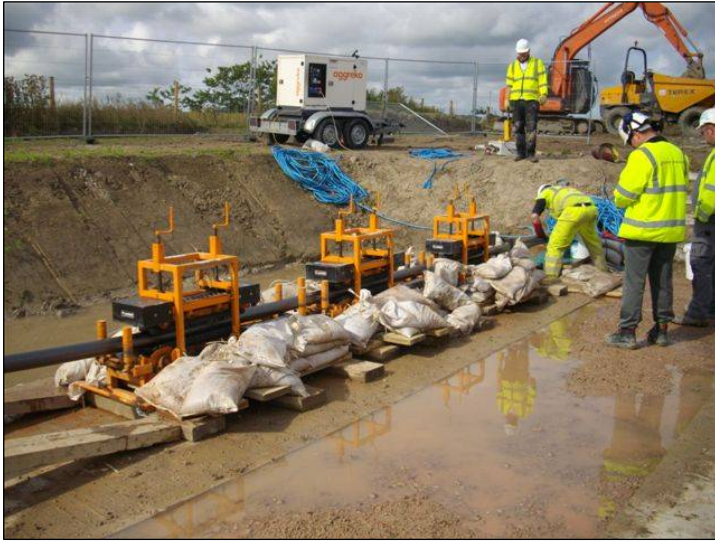
Plate 2 – Jointing pit Layout and Cable Pulling (Photo Courtesy of Prysmian)
