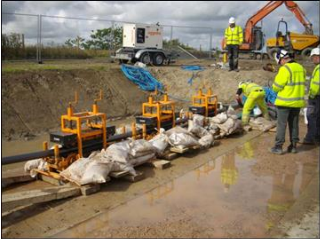
Figure 8 Jointing bay Layout and Cable Pulling. 1
