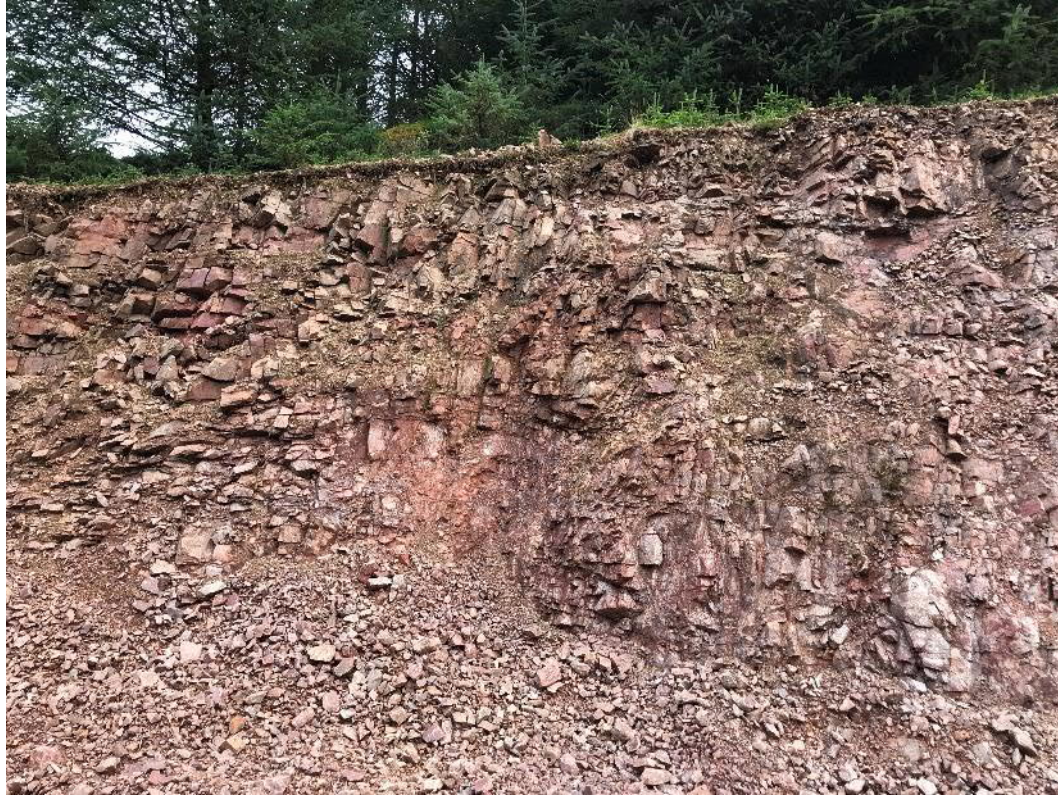
Photograph 5. Cut wall in existing borrow pit at BP03 (facing south, from NGR 399386, 6124137)
