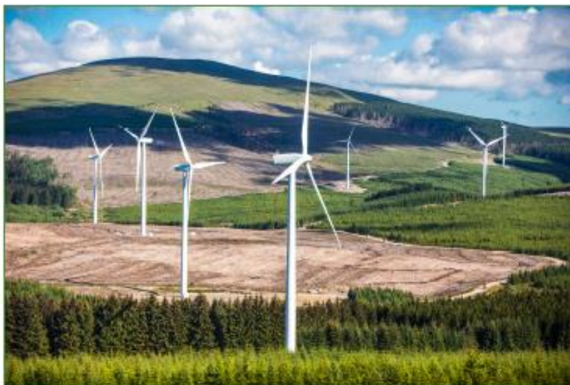
Keshmone Windfarm, turbine tip height up to 171.3m
