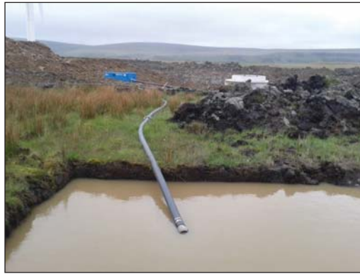
Plate 6: Typical 'Siltbuster' and settlement lagoon
