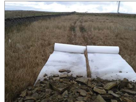
Plate 13: semi-permeable geotextile layer
