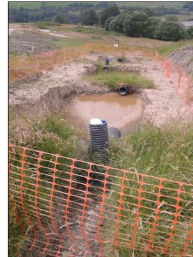
Plate 5: Typical lagoon and flocculent station
