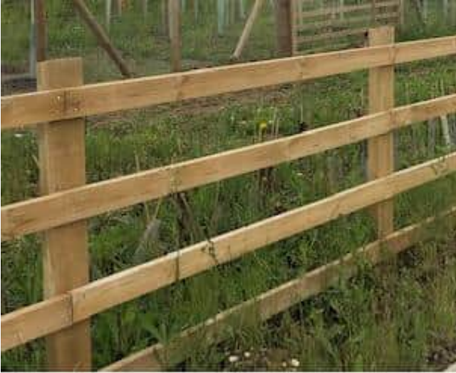
66. Figure 6-5 Example Post and Rail Fencing
