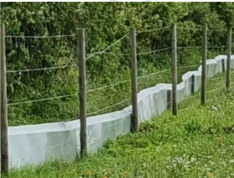
Figure 6-4 Example Post and Wire Fencing (with newt fencing behind)
