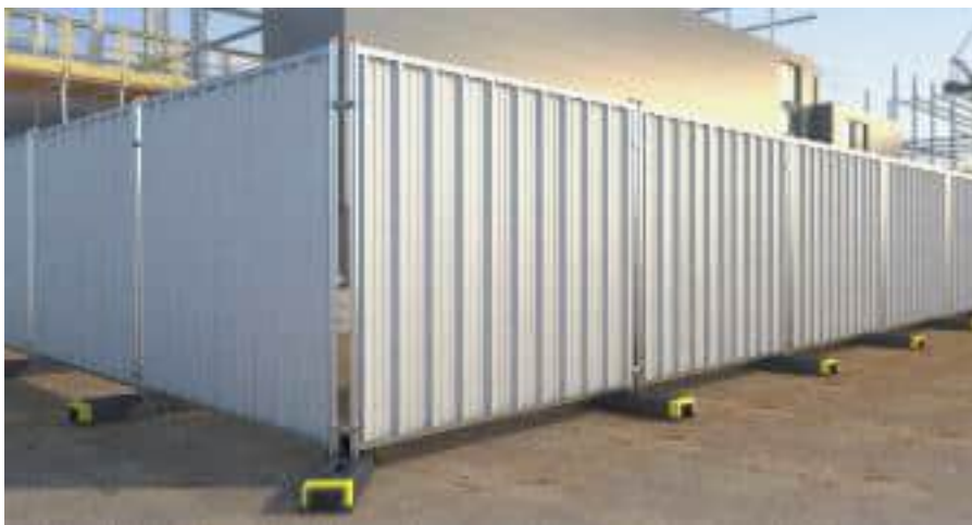
Figure 6-1 Example Metal Hoarding
