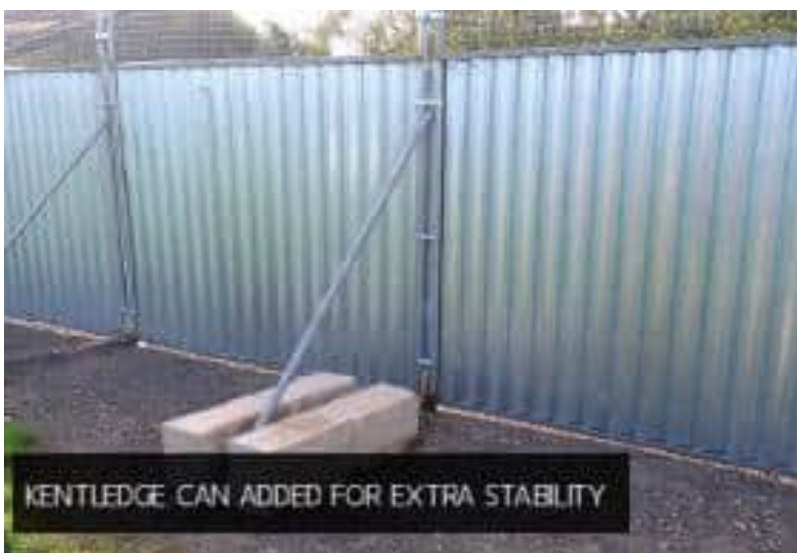
Figure 6-2 Example of Metal Hoarding Additional Support
