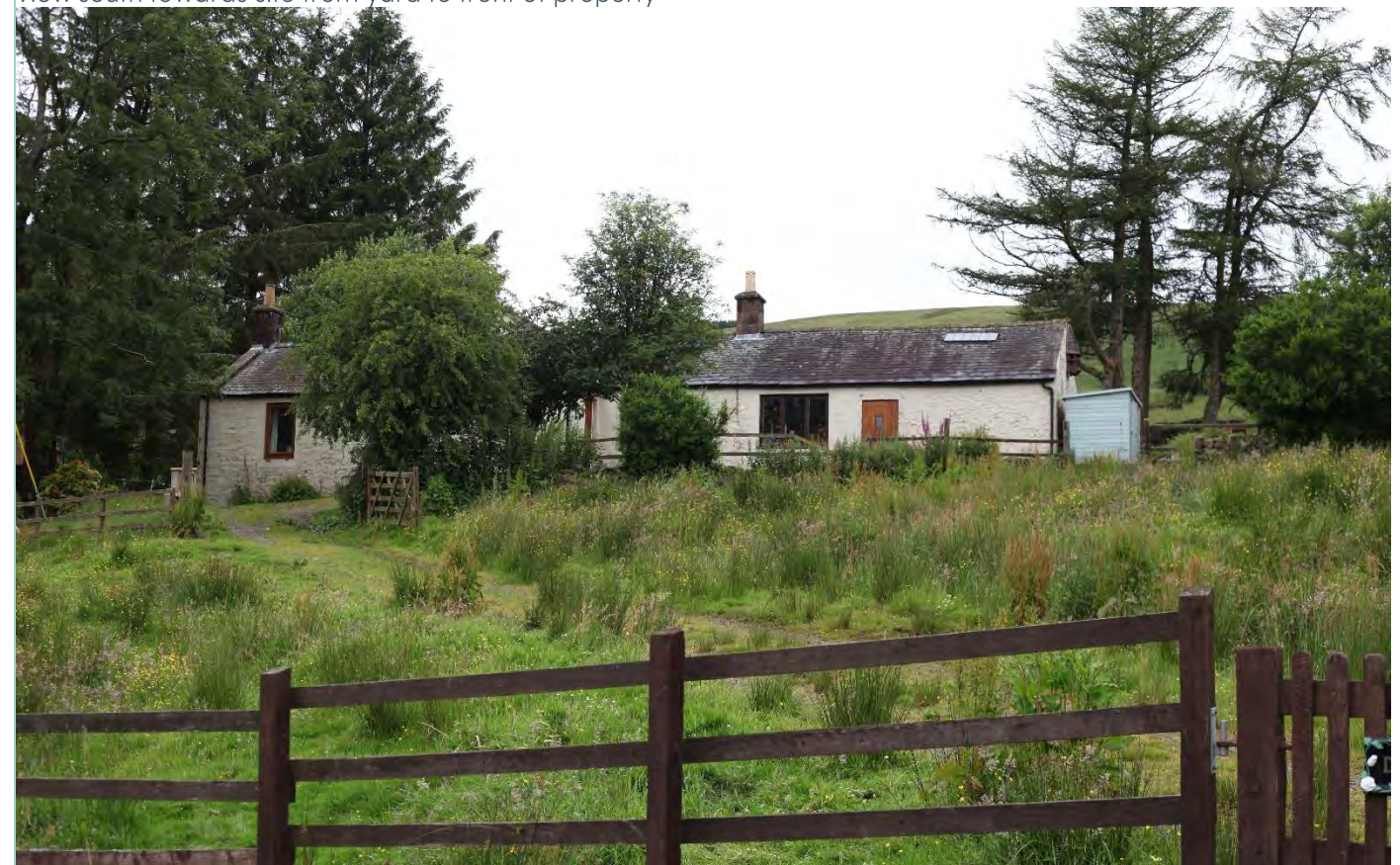
View of gardens and south east facing elevation from road
