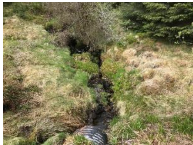
Graystone Burn - upstream of existing crossing
