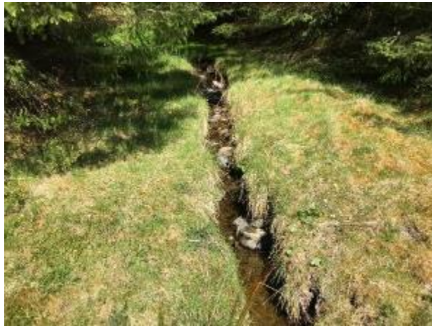
Slot Burn - upstream of existing crossing
