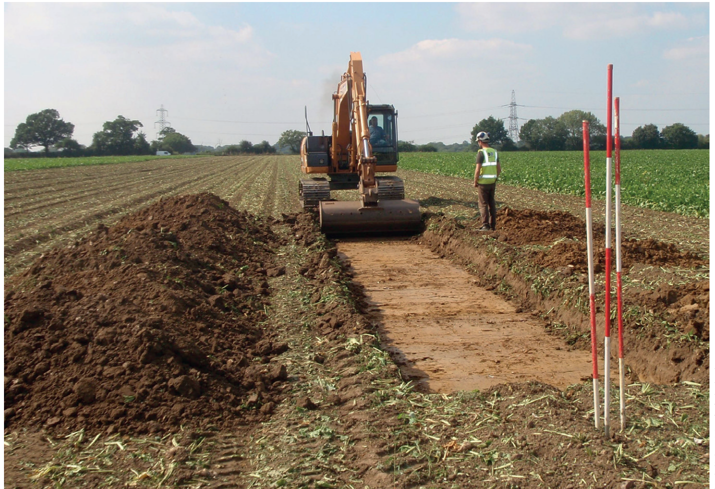
An excavator digging a trial trench.
