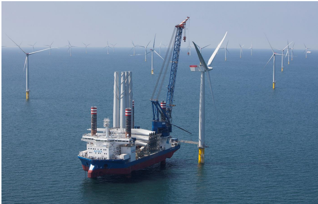
Plate 2.5 Wind Turbine under Construction (photo taken from West of Duddon Sands offshore windfarm)
