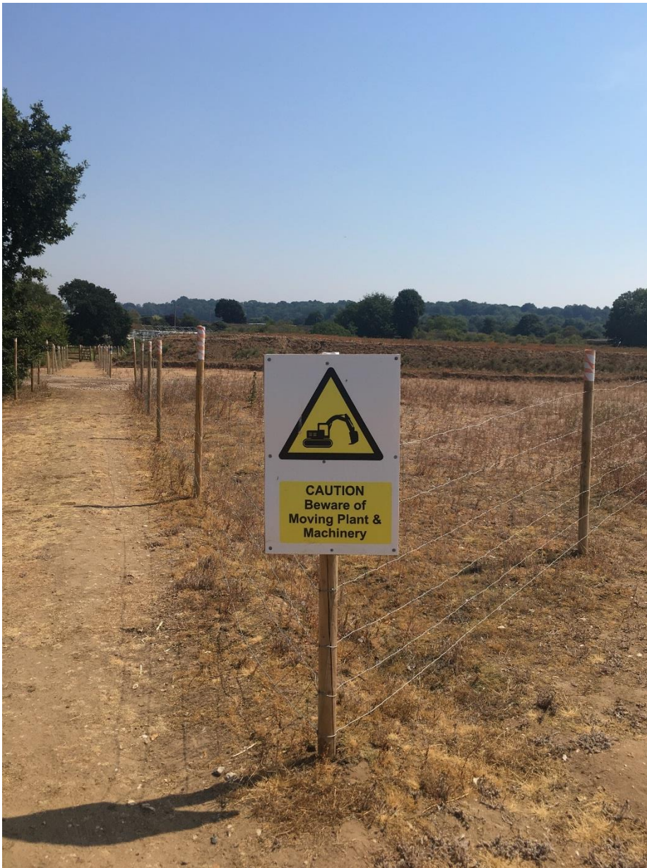
Plate 2.6 Example of a temporary fence used to delineate the boundary of the cable route working width (image taken from East Anglia ONE project)
