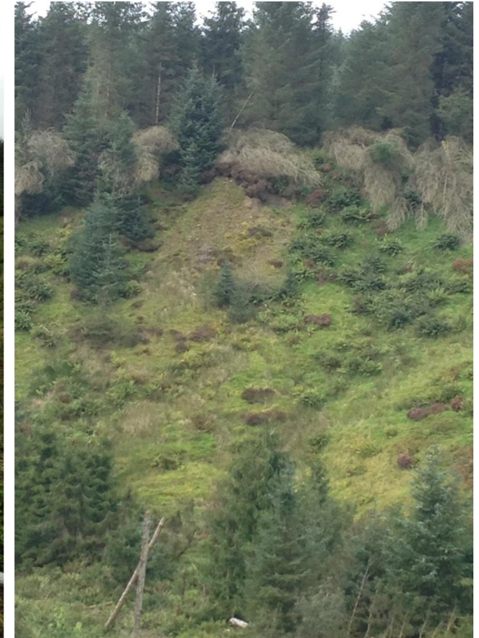
Photograph 6.4: View west towards eroding channel bank of the Glenkiln Burn, from NGR 301909, 593478
