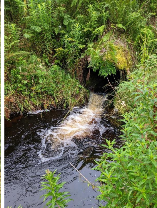
4. Culvert downstream of survey area on Clachanbirnie Burn
