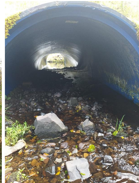
23. Pipe-arch culvert with intact instream substrate at Auchencaigroch Burn
