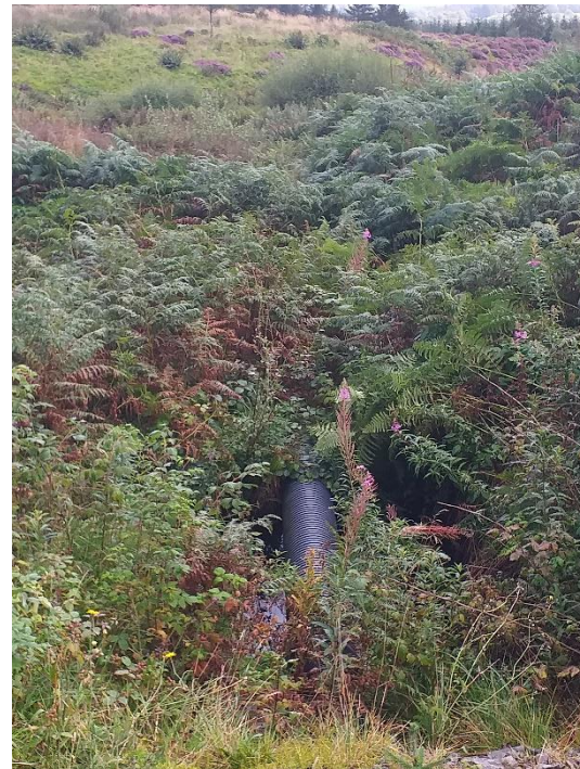
21. Small perched culvert spanning the forestry track at Torr Linn
