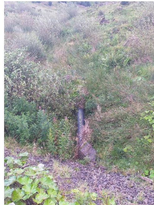
18. Small perched culvert spanning the forestry track at Cat Cleugh
