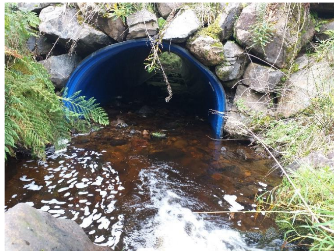
16. Pipe-arch culvert with intact instream substrate at Blenoch Burn
