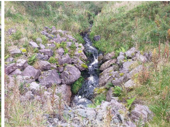
27. Upstream of culvert on Shiel Cleugh
