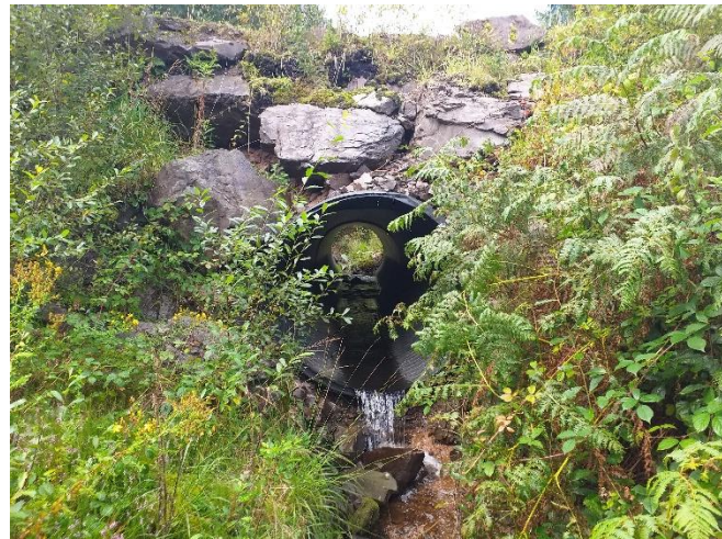
20. Culvert spanning Black Linn at forestry track
