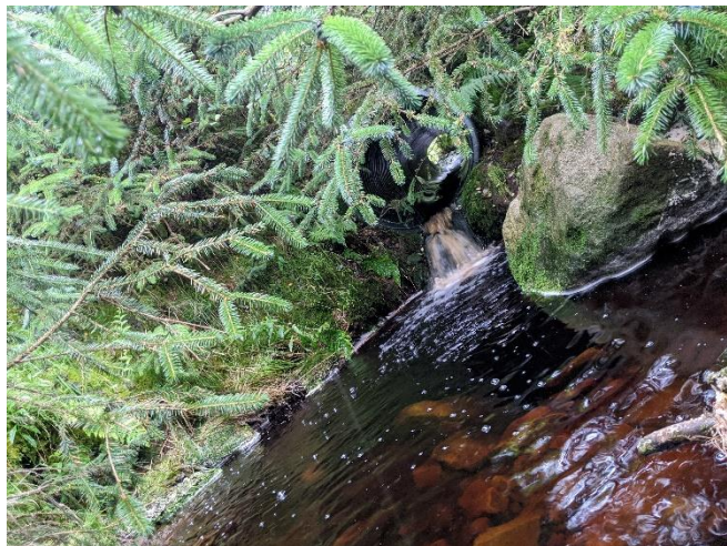
6. Culvert downstream of survey area on Yellowtree Grain
