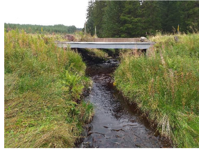
14. Deer burn crossed by two clear span structures
