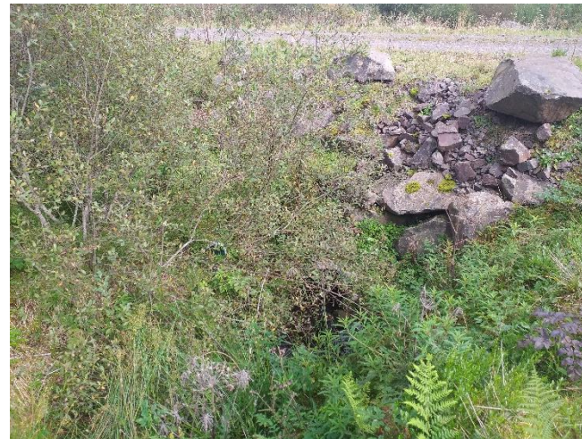
26. Pipe culvert under forestry track at Auchendowal Sike
