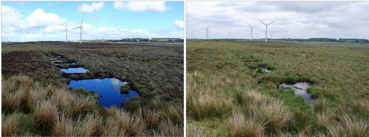
Photos 1 & 2: Area of wave damming at Black Law windfarm immediately following treatment (left) and two years post treatment (right)
