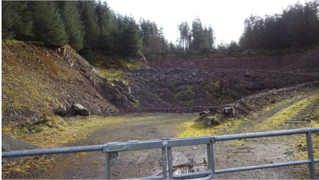
Photograph 10.3.1: View from the base of the existing borrow pit looking up the back wall, taken at 29524 59410 looking south east.
